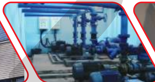
MAINTENANCE POMPA TRANSFER
